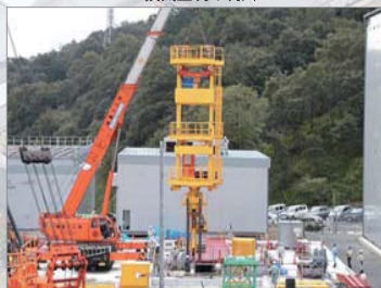
換気立坑へのスcaffoldingの設置
